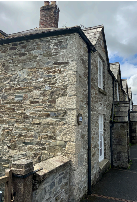
• Parkwood Cottage (render removed)
