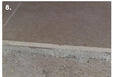
1. excavation 2. pour foam glass on breather membrane 3. spreading 4. tamping to compact & level 5. breather membrane 6. tamping limecrete slab 7. edge cork strip 8. tiling onto lime slab
