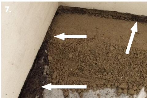
1. excavation 2. pour foam glass on breather membrane 3. spreading 4. tamping to compact & level 5. breather membrane 6. tamping limecrete slab 7. edge cork strip 8. tiling onto lime slab
